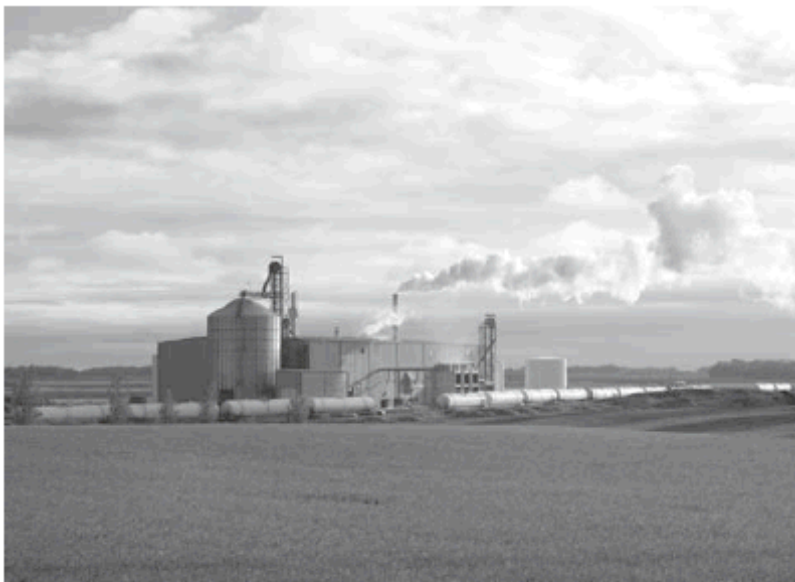
Ethanol production plant utilizing corn as a feed stock, located in South Dakota
